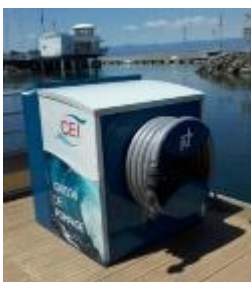
Figure 36 : Station de pompage fixes
